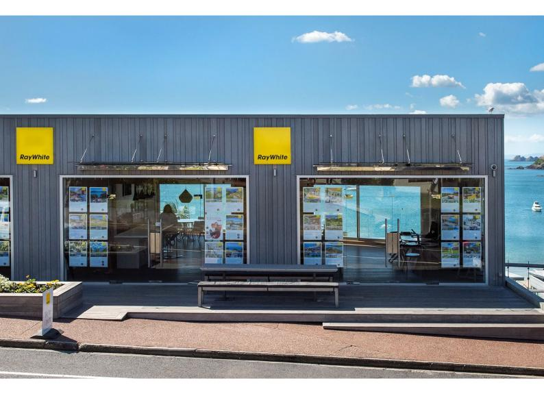
Ray White on Ocean View Road, Waiheke Island, is exposed to a lot of direct sunlight and salty sea-spray. For their refurbishment, WOCA Exterior Oil was chosen to protect and enhance the cedar cladding. The surface was first cleaned and prepared with WOCA Exterior Cleaner, which removed all the silvered dead timber and what remained of the existing finish. This created a fresh timber surface, ready for the Exterior Oil.
